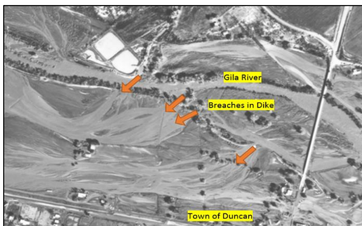
Figure 2.2-Aerial photo of the 1978 Duncan flood [6]
